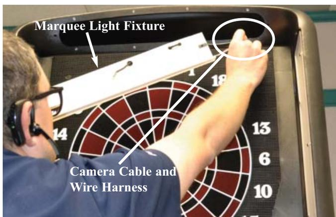
14. Insert both the Camera Cable and Marquee Power Harness through the opening for the marquee.
