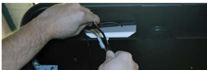
15. Using the Access Hatch we opened in step 9, feed the rest of the cabling and wires down the side of the machine.
